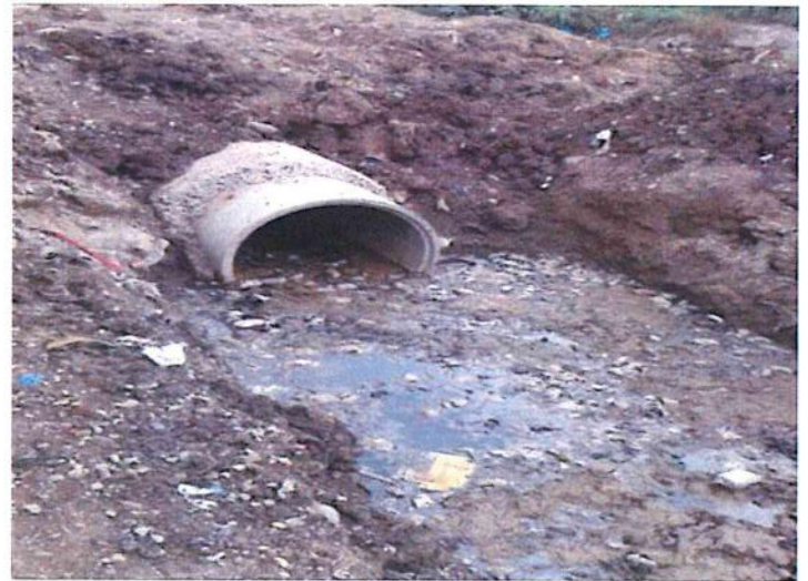
Plate 2: Incomplete section of Sewer Blue Estate, Nairobi
