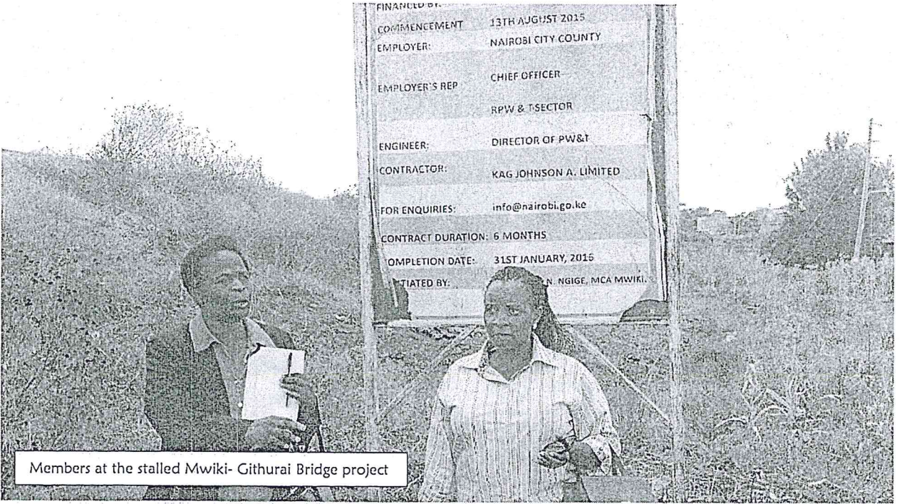
A section of stalled Mwiki-Githurai Bridge project
