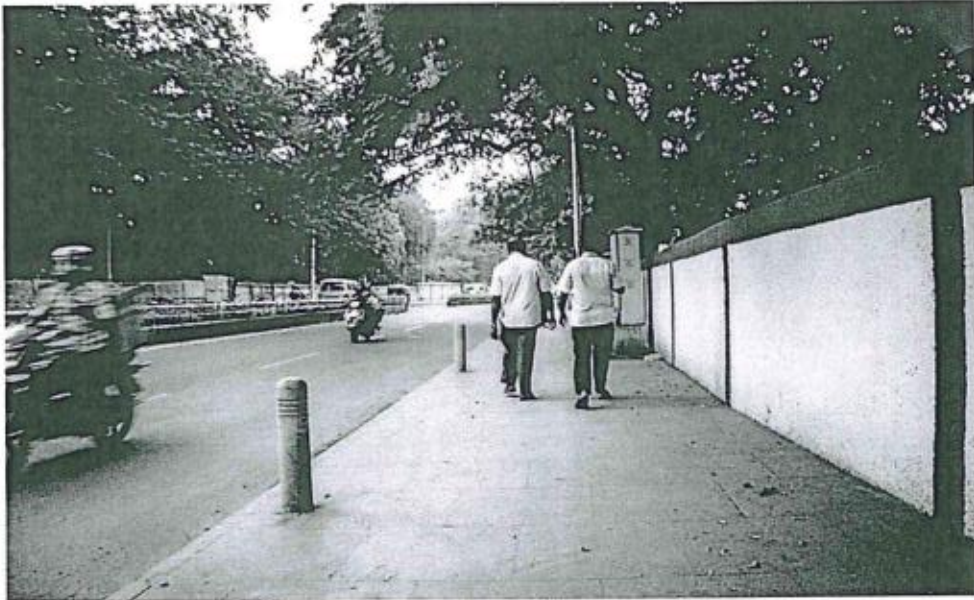
The same road in Chennai India after NMT construction
